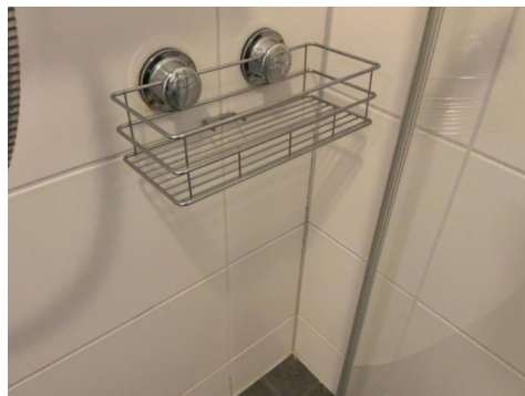
Sprekker i mykfuge
